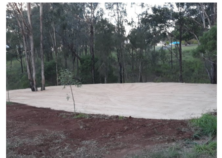
Have you been wondering what this is? It's the site of the Proston Labyrinth which has been prepped and is ready for the pavers to be laid. Thanks to Heath Sanders of Sanders Bobcat & Mini Excavator Hire for his efforts.
