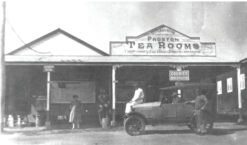
Left: Proston's first commercial building, Proston Tea Rooms and Post Office, Rodney Street.
